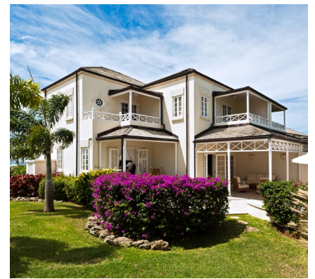
Apes Hill Villas Apes Hill, Barbados
